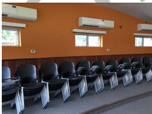
Figure 6: Three Back of the Room Windows Open (Trial 2)
