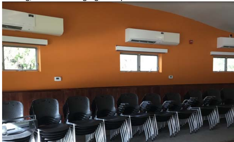
Figure 3: Assembly Room Back Wall Fan Coil Units
